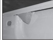
c) Then push and compress foam into box cavity a little at a time.
