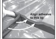
c) Continue applying seal to lip along bed floor following up and down the ribs. Use firm pressure. Continue on stopping at mark on opposite side.
