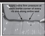
d) Continue around corner . At floor, leave protective backing to wall side. Work across floor with firm pressure up and down each rib. Then peel backing off wall side and apply pressure to it. Next continue with both seals up box. Stop at box contour near top. Leave adhesive protectors on- mark and cut seal to length for top and V-cut - as at top of other side -then finish adhering.
